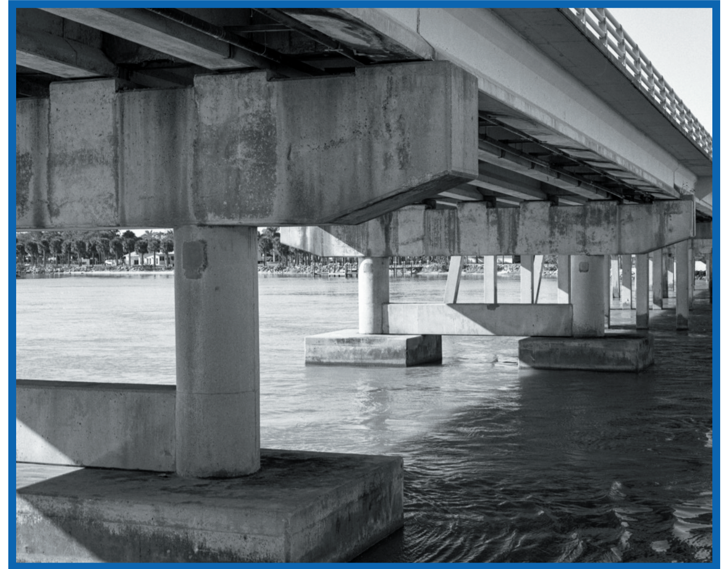
Fort Pierce South Bridge—Colin Knight
